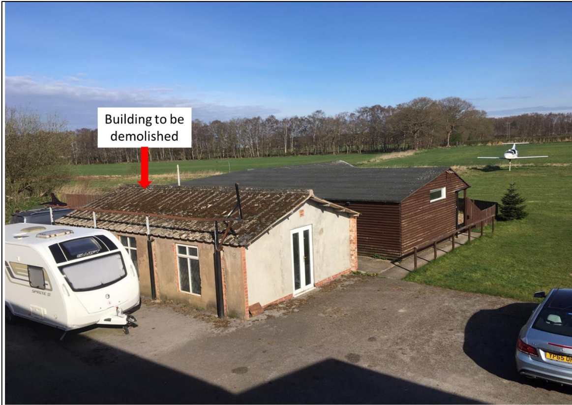
View north of the existing building to be demolished
